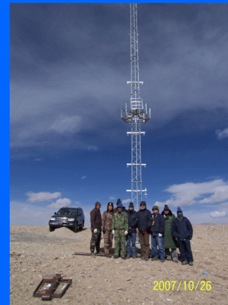
CT2 sensors on 40m tower
